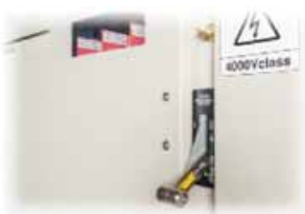
A convenient isolation switch kills the main power to the VFD to allow for safe servicing.
