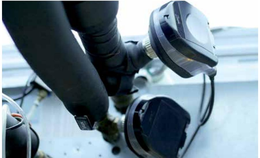
*NovoCon® actuator in combination with AB-QM valve*
