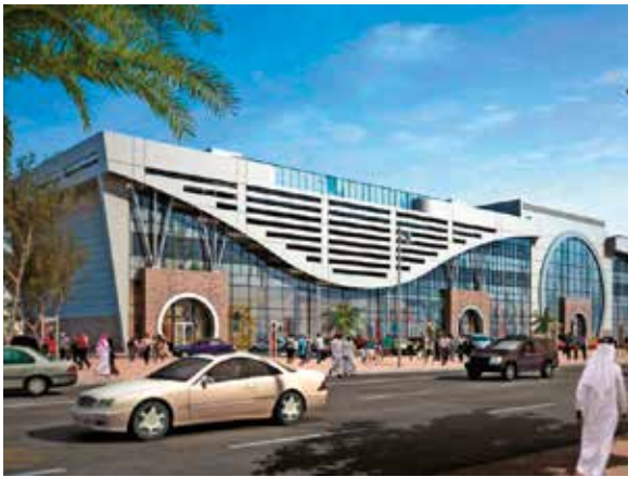
Location: Doha, Qatar Project: Barwa Commercial Avenue Application: AB-QM for cooling
